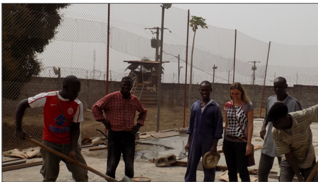
Federica supervises the workers (UNV programme, 2016)
